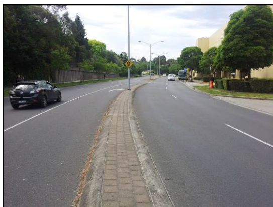
Figure 7: Snedden Dr - View North adjacent Subject Site
