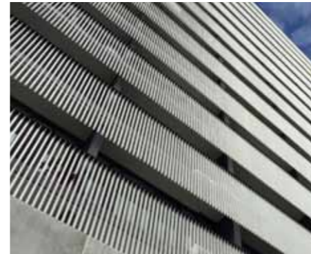
Metal Screening Residential Tower 1
