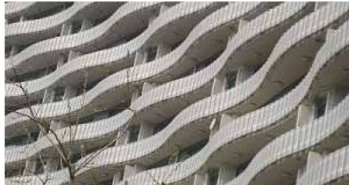
Metal Screening Residential Tower 1
