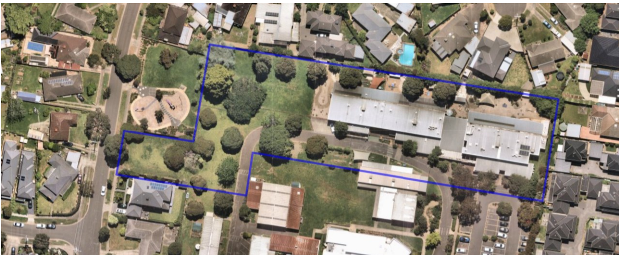
Figure 4 – Aerial view of the child care centre.
