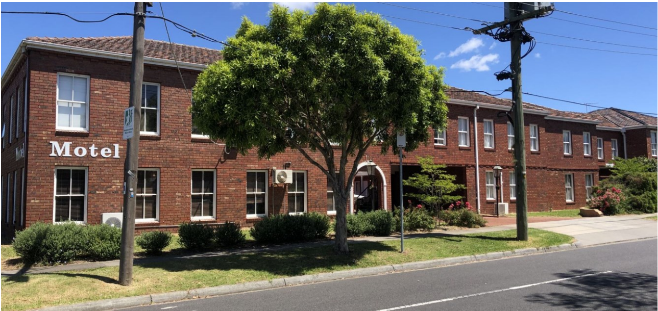
Picture 3 – No. 11-17 Kerferd Street taken from the corner of Ferntree Gully Road and Kerferd Street.
