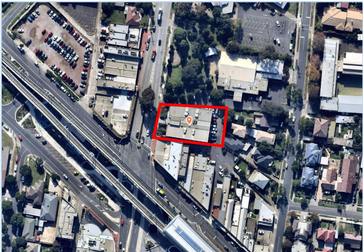
Figure 1: Aerial view of the site at 270 Clayton Road, showing the approximate site boundary. (Source: Nearmap, Mark-up: WRAP Engineering)
