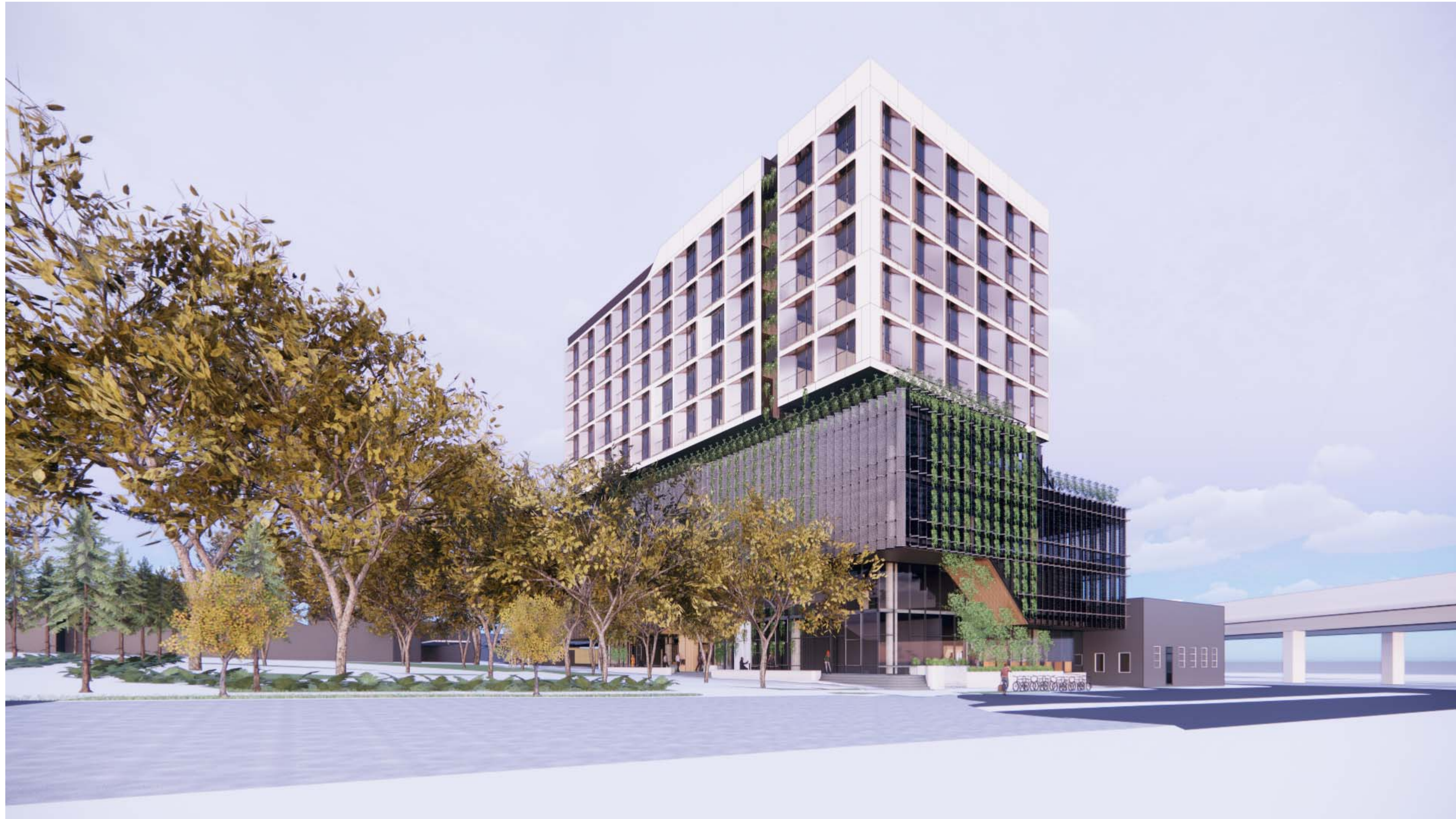
270 CLAYTON ROAD, CLAYTON
