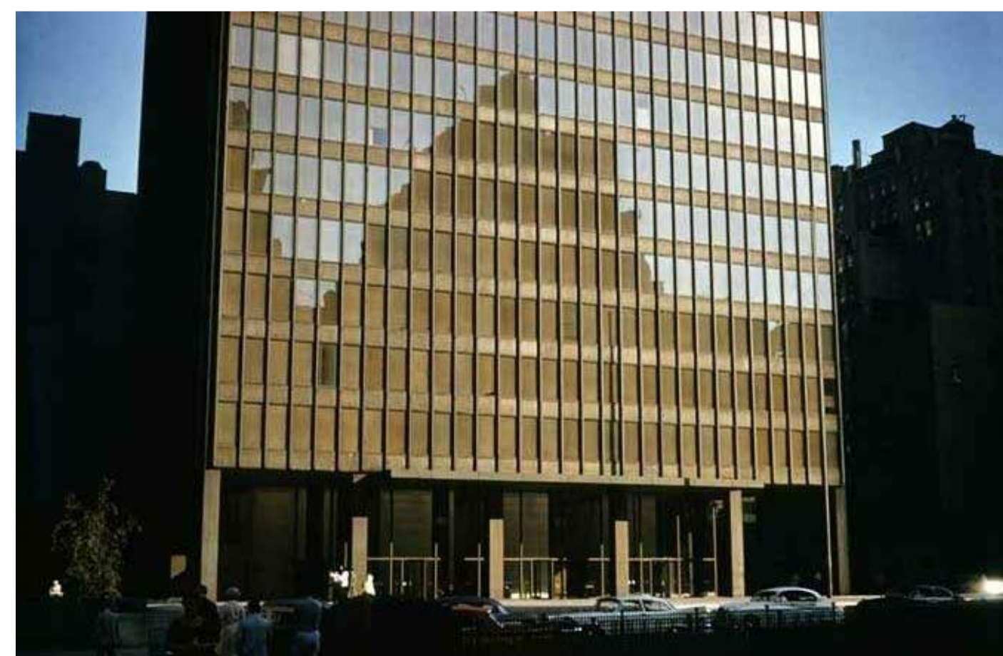
GL04 BRONZE GLAZING IN ALUMINIUM FRAMES. ANODISED FINISH - SATIN LIGHT BRONZE
