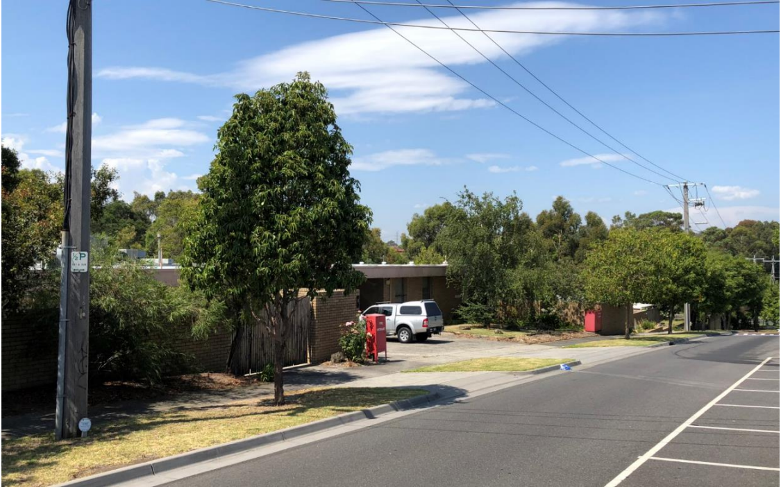
Figure 3. 1-9 Allen Street (pre-demolition).
