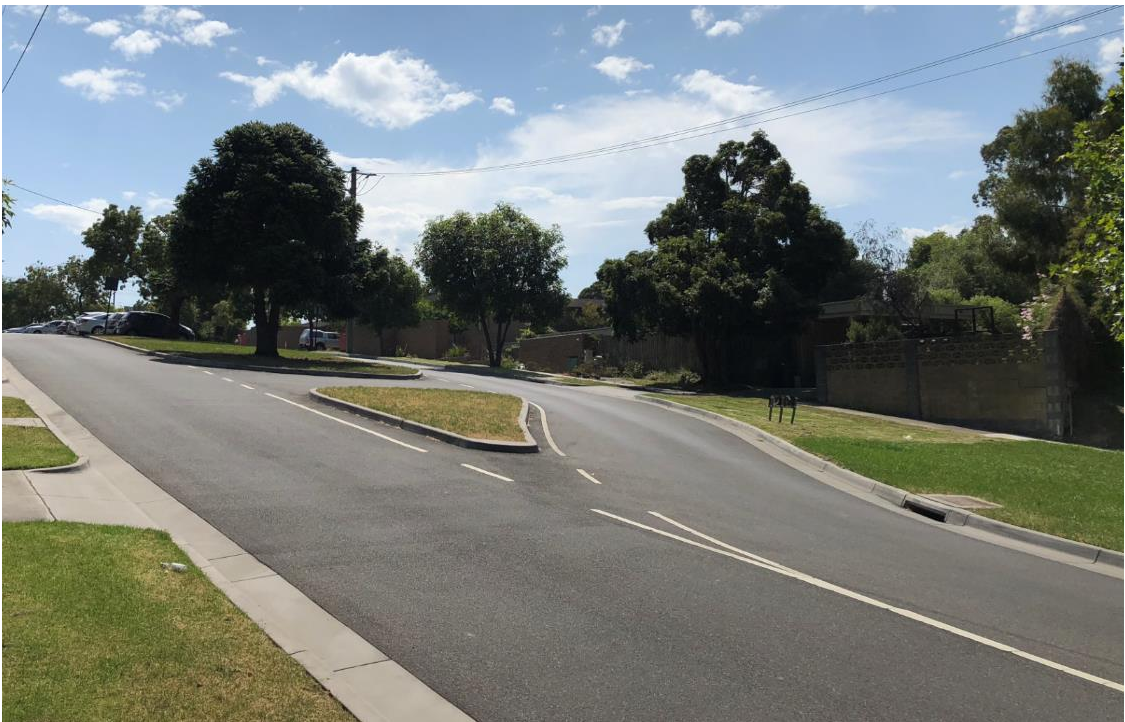
Figure 4. 1-9 Allen Street (pre-demolition).
