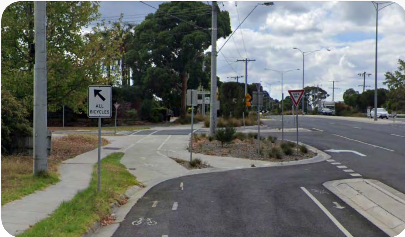
Figure 24. Example of cycle path cut through at street intersection Stud Road, Wantirna
