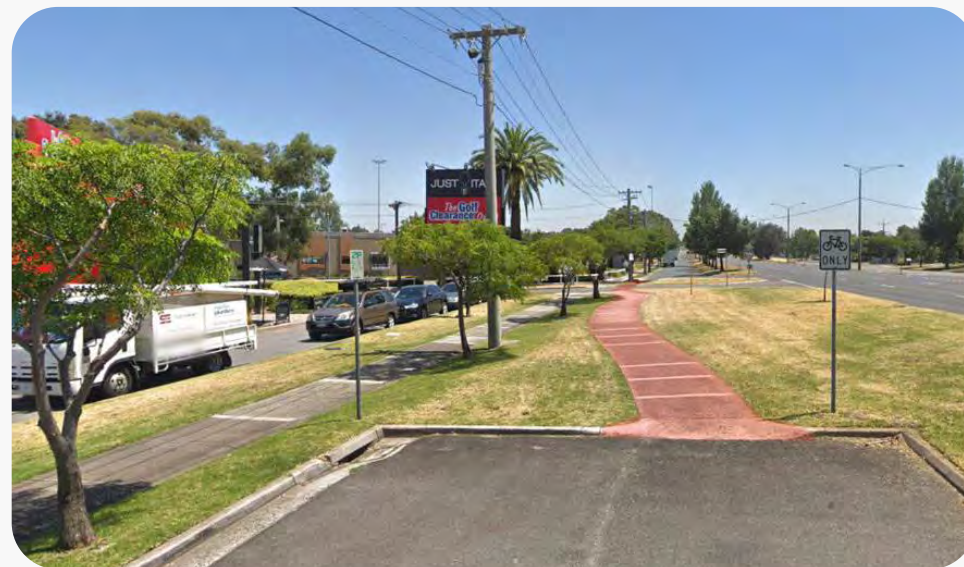
Figure 16. Example of cycle cut through on Dandenong Road, Oakleigh East.
