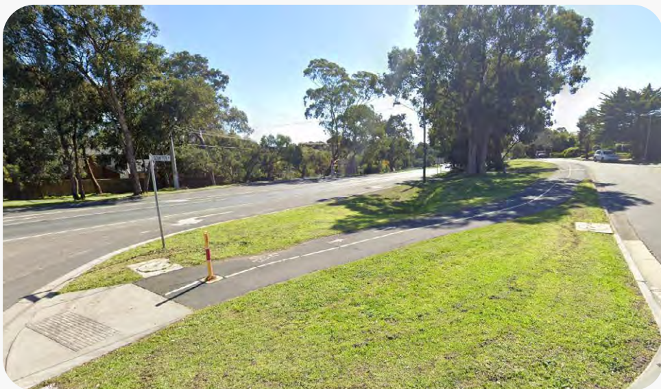
Figure 15. Example of cycle path within outer separator at Andersons Creek Rd in Doncaster East.
