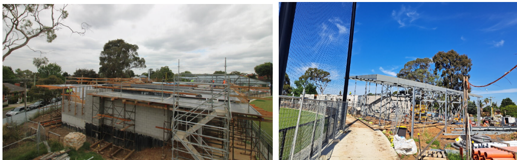
Images of the new pavilion at Mount Waverley Reserve
