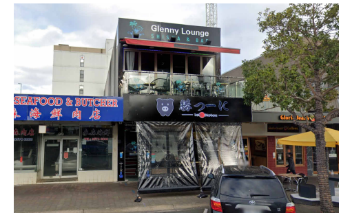
99 KINGSWAY GLEN WAVERLEY, VIC 3150 DOUBLE STOREY RESTAURANT
