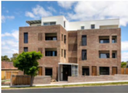
Aboriginal Housing Victoria Developer: Aboriginal Housing Victoria Architect: Breathe Architecture
