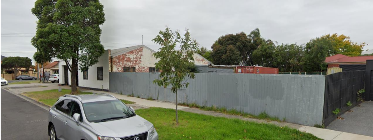
Existing building presenting to Bowen Street
