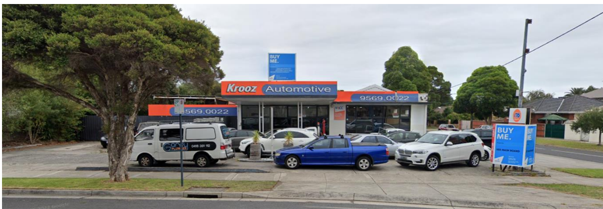
Existing building presenting to Kangaroo Road
