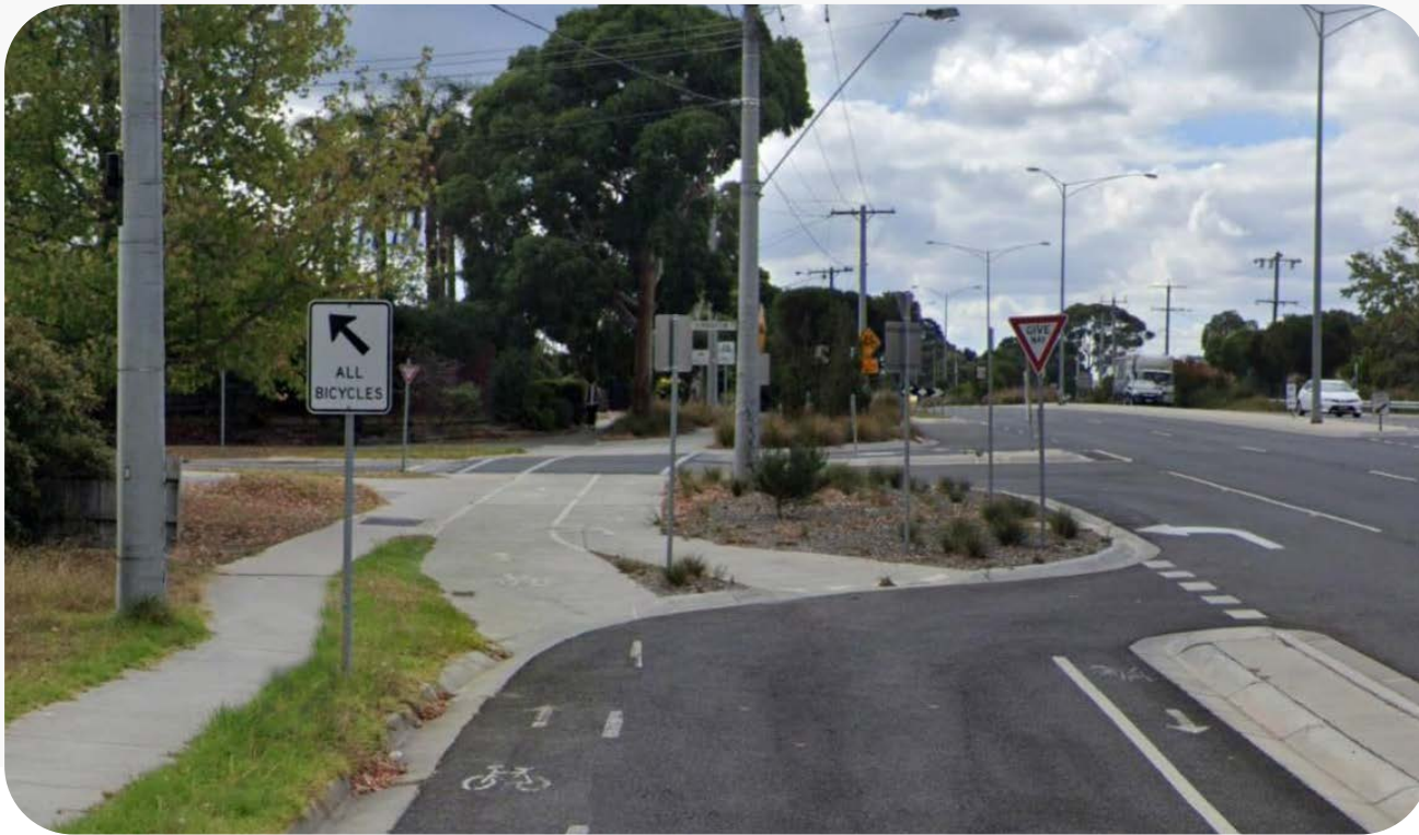
Figure 24. Example of cycle path cut through at street intersection Stud Road, Wantirna
