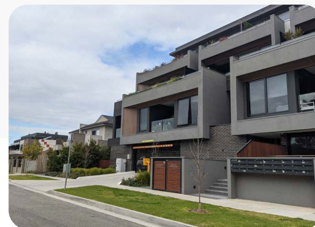
Example of poor street interface dominated by services and car park entry
