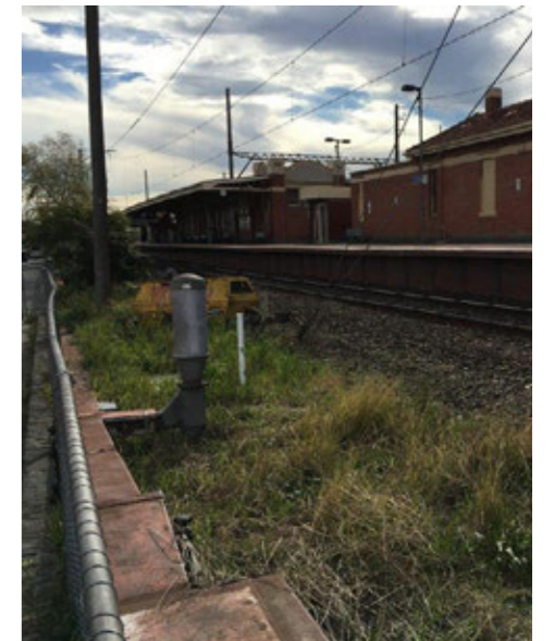
Figure 25 Oakleigh third track Remove the redundant third track to provide direct access to the platform and space for a new Shared Use Path.
