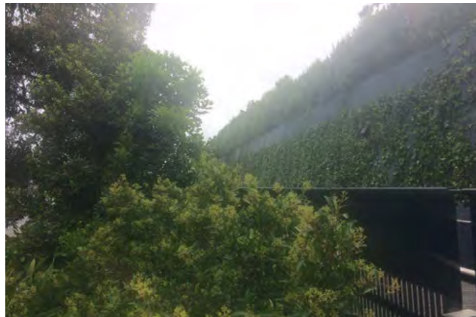
Figure 13 Vertical planting on a mesh structure, with layered landscape elements in front planted into natural soil, Melbourne Park Eastern Plaza (Jackson Architecture)
