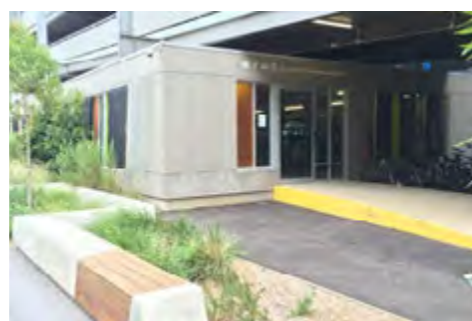
Figure 6 Integrated end of trip facilities, Monash University Clayton Campus
