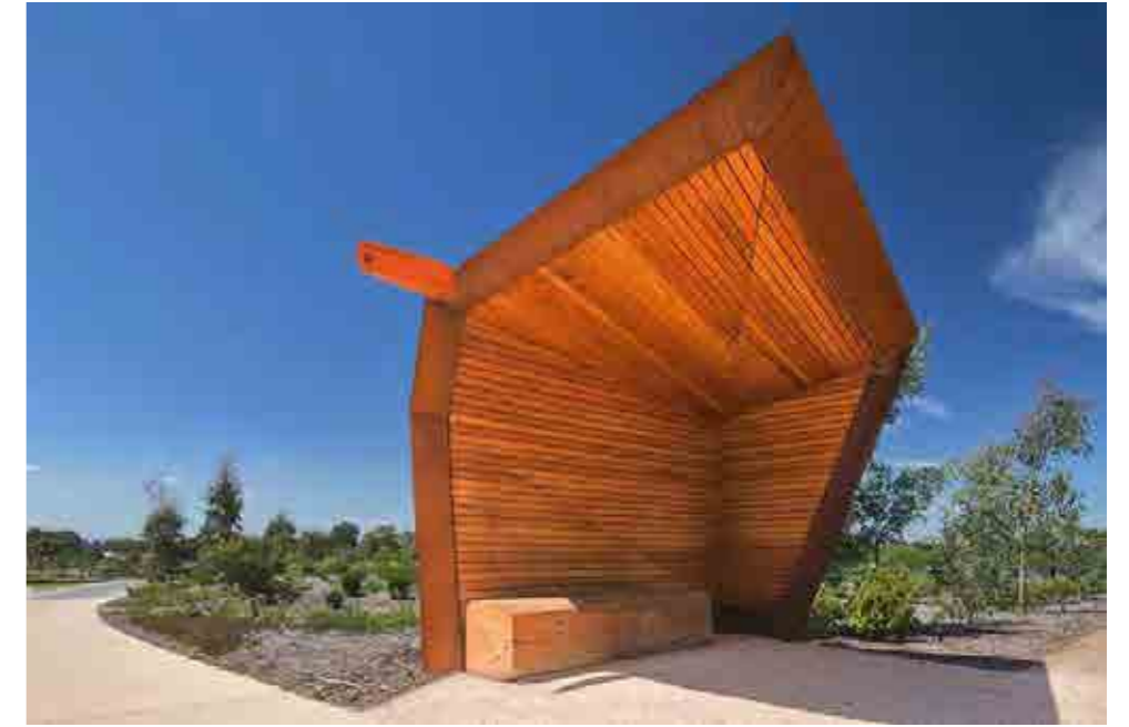
Figure 48 Distinctive but sensitive rest stop, Australian Shelter Gardens (BKK Architects) Image : John Gollings
