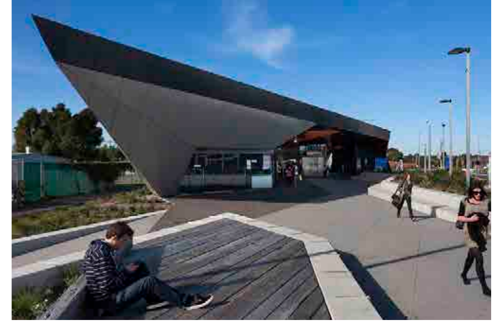
Figure 60 Integrated kiosk and station facilities, South Morang Train Line (COX Architects) Image : Dianna Snape
