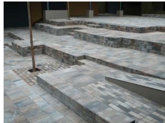
Step designs for seating & access: Limoner Square in Spain by EMF
