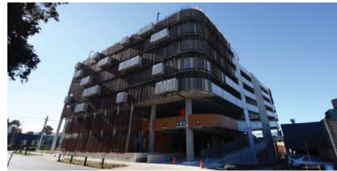
Euneva Community Health and Multi Level Carpark, 2012
